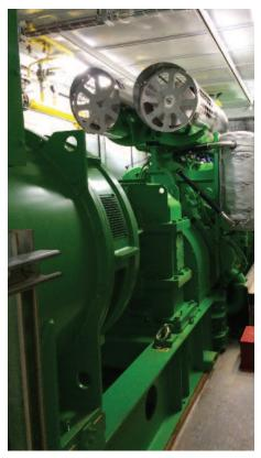
Figure 2 - Natural Gas Fired Generator Set
