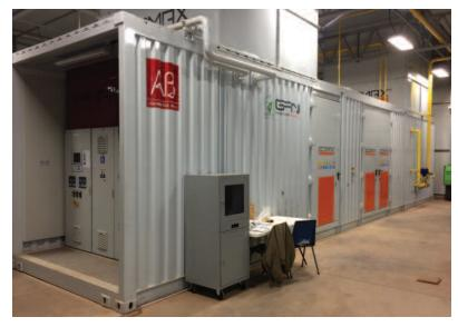
Figure 3 – Engine House for Figure 2 in a Modified Shipping Container
